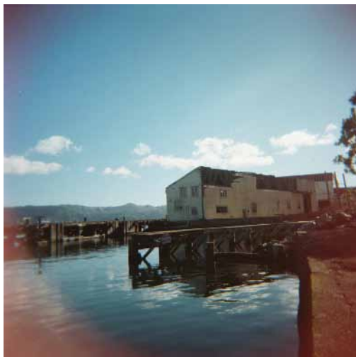
Figure 2 Shipwright building - Shelley Bay, Wellington.
