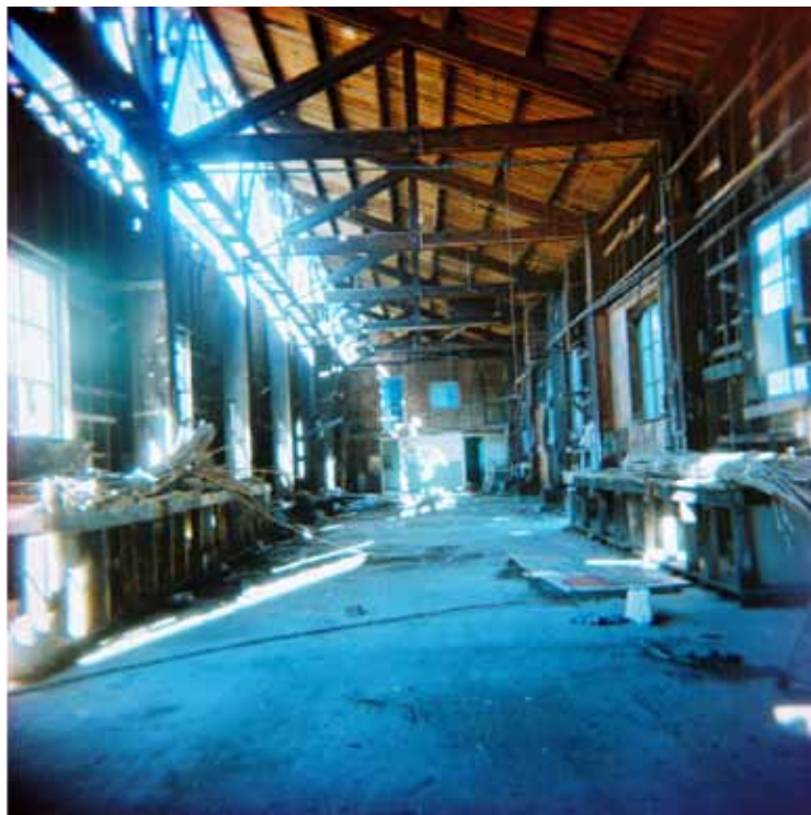
Figure 4 Interior of Shipwright Building
