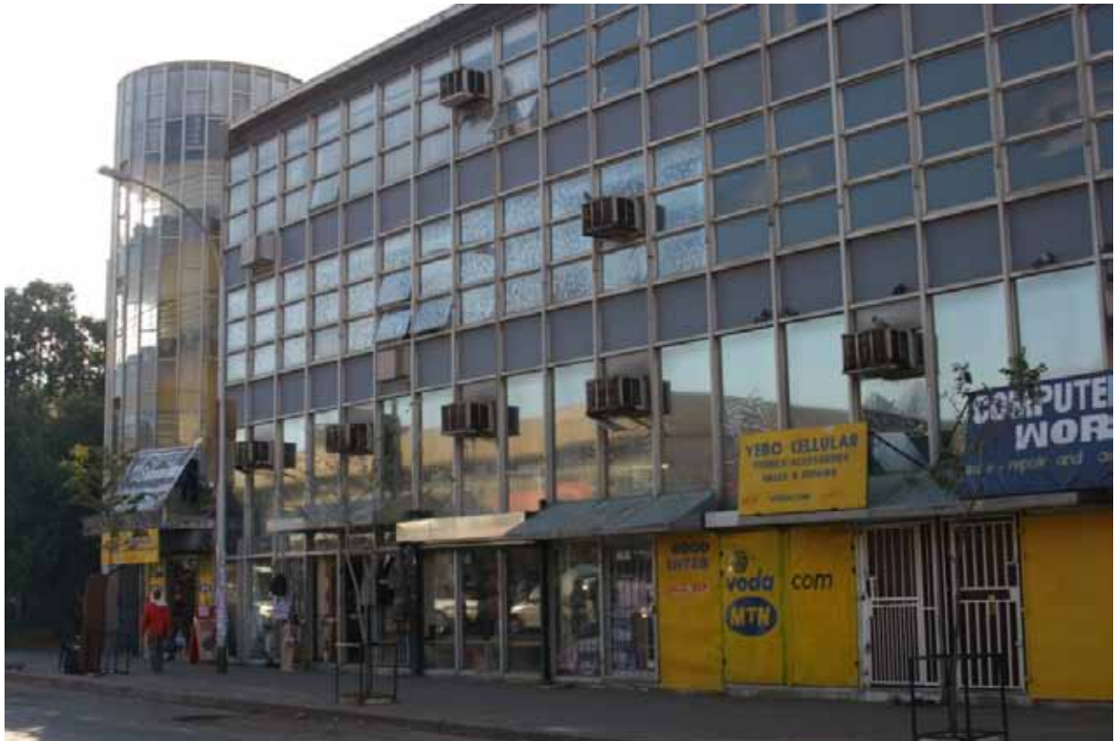
Figure 10 Roodepoort Bank, South Façade, 2011.
