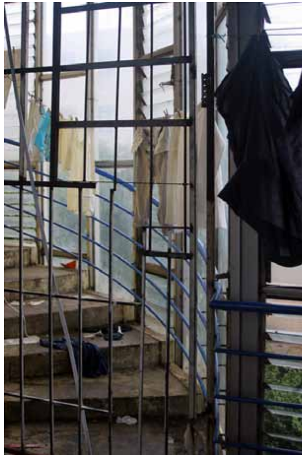
Figure 14 Roodepoort Bank, December 2010.
