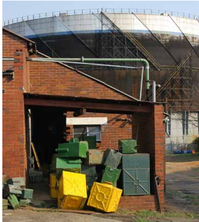
Figure 7 Gas Tank with old gas meters 2011.
