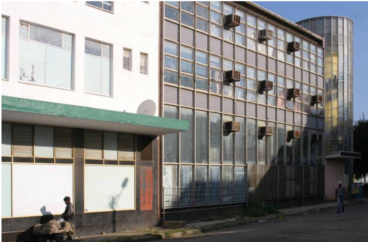
Figure 12 Roodepoort Bank, North Façade, 2011.
