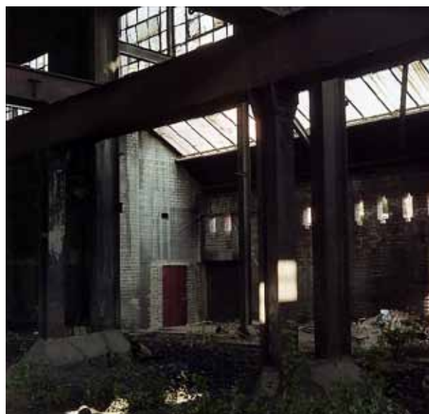
Figure 4 Interior, Gas Works 2011.
