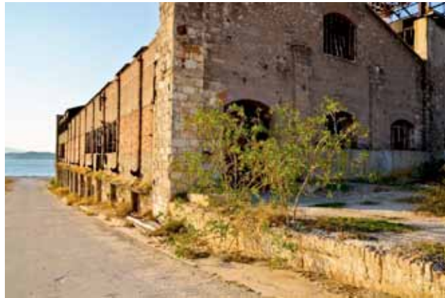
Figure 4 The Factory of Fertilizers in Drapetsona area, exterior view.
