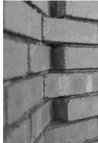
Figure 14 Obtuse corner in open brick bonding (photo: Roger Jardine).
