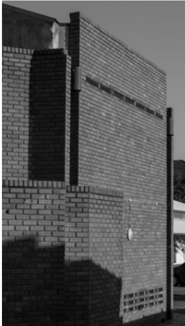
Figure 11 Diaphragm wall facing north-west. Note fresh air inlets by way of the perforated brickwork at the bottom and the outlet at the top (photo: Roger Jardine).
