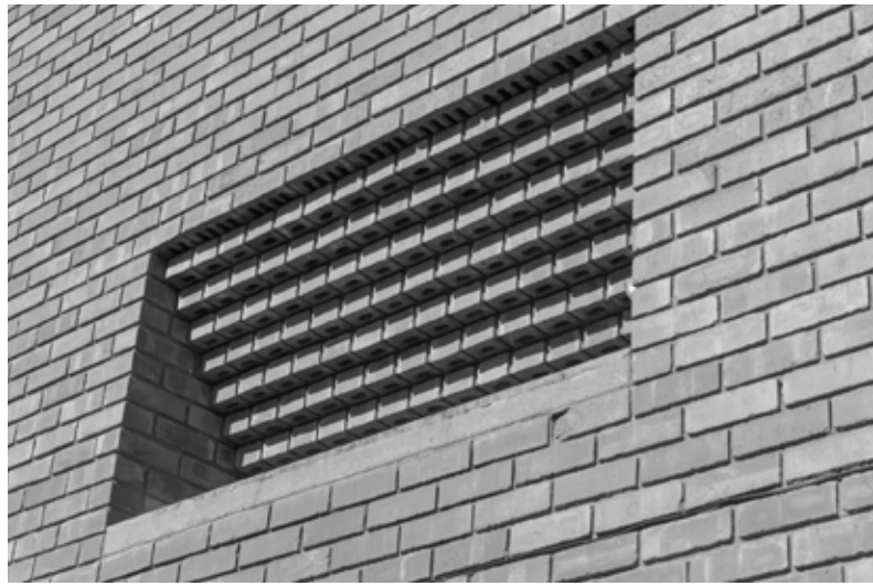
Figure 7 External corbelling to illuminate the altar (photo: Roger Jardine).
