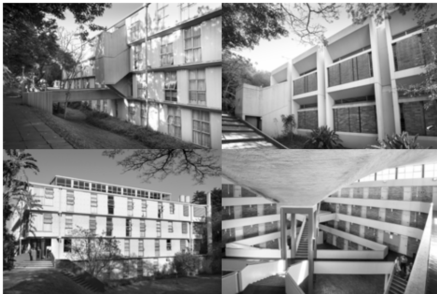
Figure 3 John Bews (female) residence, 1964; Scully (dining) Hall, 1965; and Mabel Palmer (male) residence, 1966, exterior and interior, Howard College campus, UKZN, Durban. Hallen & Dibb Architects (photo: Angela Buckland).
