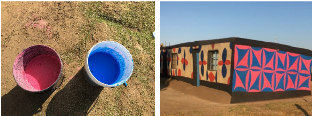
Figures 9 and 10 An example of morella distemper stabilized with soft maize porridge or milk on a rural homestead, Clear Water Farm near Warden (photographs by the author).
