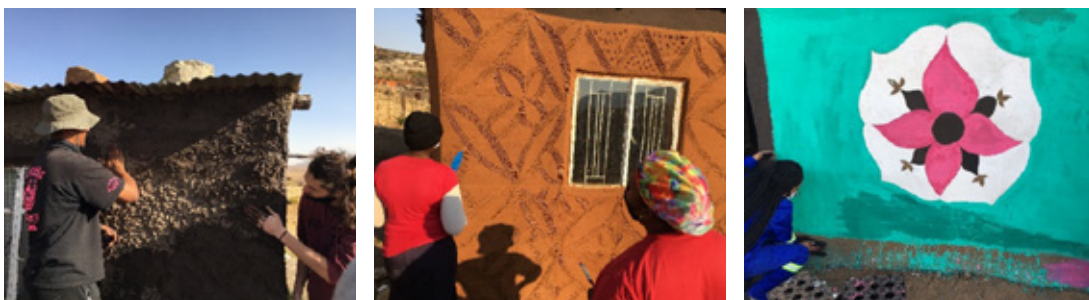
Figures 11, 12 and 13 An example of a rough layer ( parra ) to key well with the following smoother layers before litema can be designed with or without morella on the dry final layer (photographs by the author).
