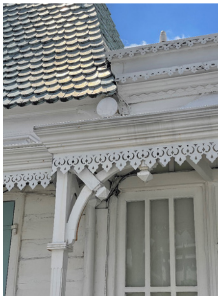
Figure 9 Roofing details of a Créole house showing the shingles, ornate lace fascia, the wooden elements. (photograph by the author, 2024).
