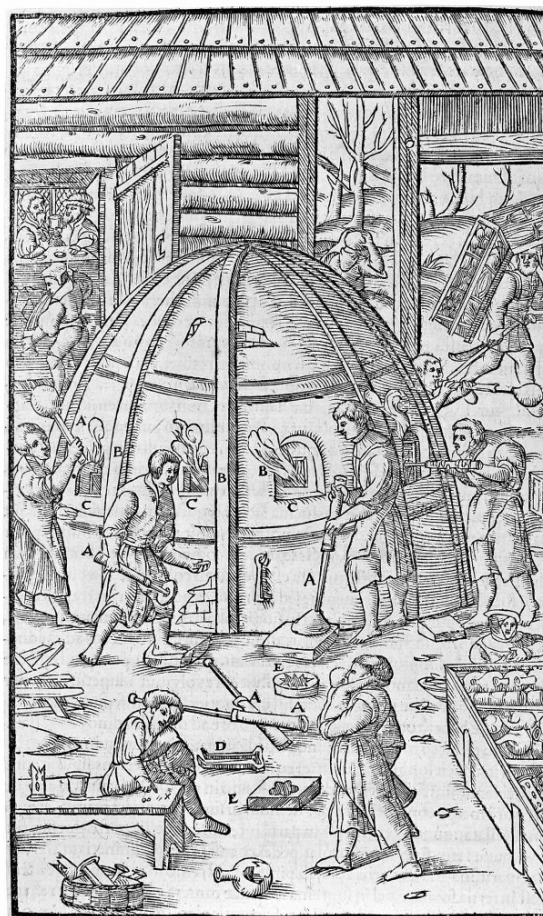
Figure 1 Glassblowing, Agricola, De re metallica . Sixteenth century (retrieved from https://www.caia.us/post/the-tools-of-america-s-first-glass-blowers ).
