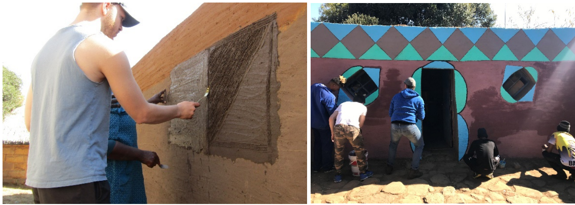
Figure 6 The SL workshop in 2024 at the Basotho Cultural Village of litema plaster applications (photographs by the author).
