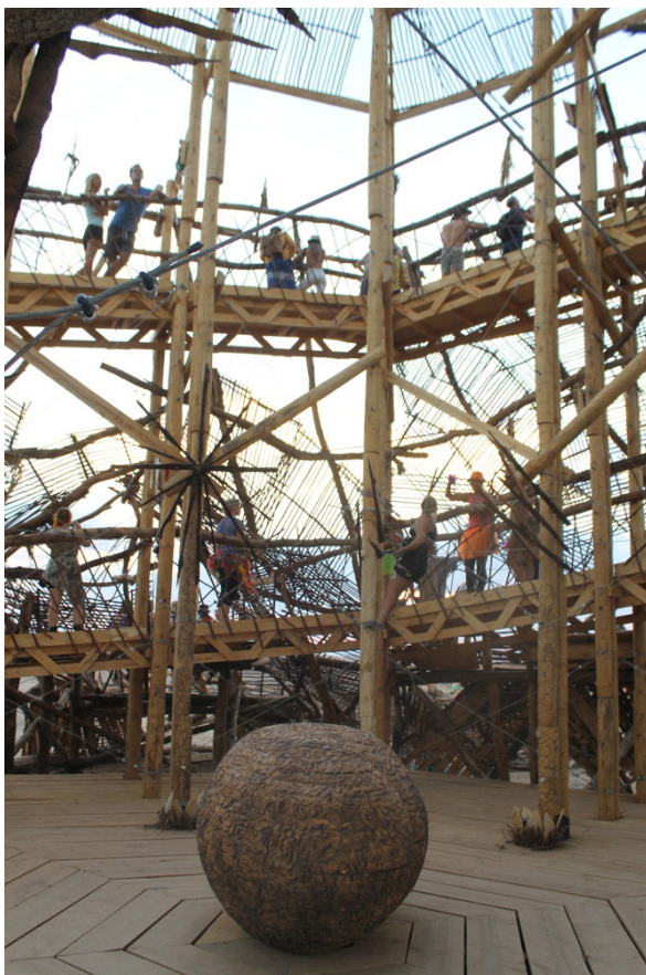
Figure 4a Structural main elements and centrally placed sculpted baobab seed (photo by John Steele).
