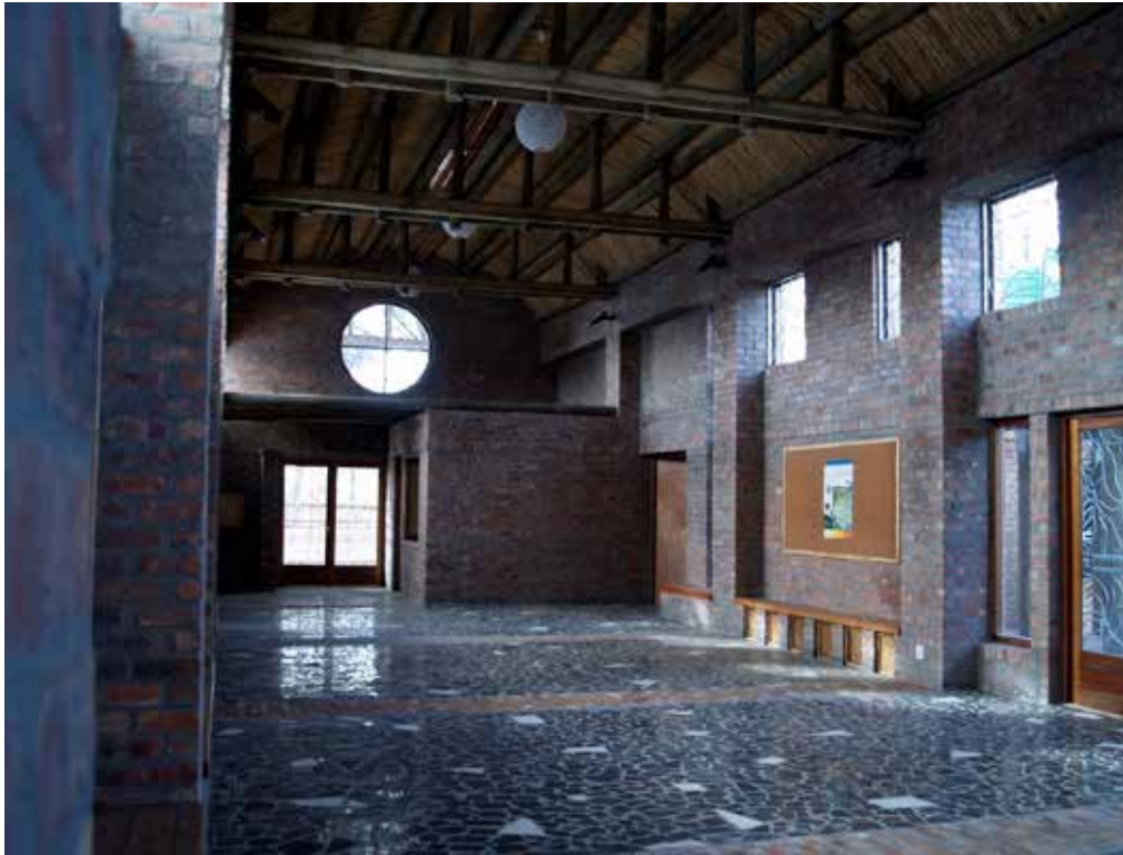
Figure 7 Tsoga, double-volume “spine”, 2004 (source: courtesy of Collis & Associates).
