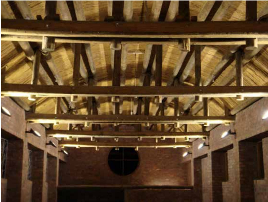
Figure 8 Tsoga, gum-pole truss and reed ceiling, 2004 (source: courtesy of Collis & Associates).
