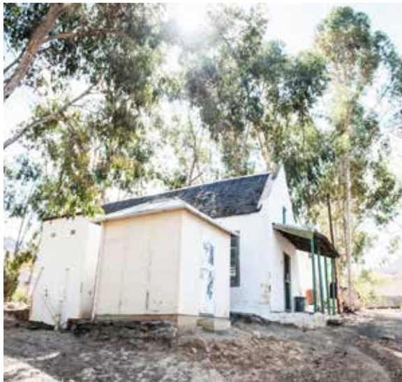
Figure 12 Existing ablation structures cladded to building in the link between the church and the shoe factory (photo from Franklin 2015).
