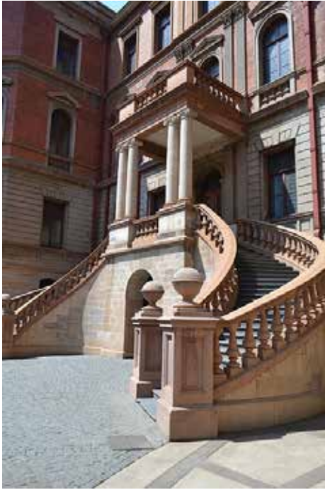
Figure 2 Ciment-fondu balusters, the Palace of Justice, Pretoria Church Square (photograph by N.J. Clarke).
